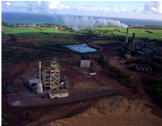
Fig. 11. Gasification plant in Maui, Hawaii, converts sugar cane to electricity (Source: Biomass Energy, 2022. Photograph courtesy Warren Gretz/NREL (National Renewable Energy Laboratory, NREL))
